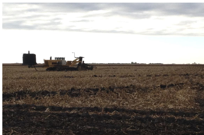
Figure 1. Subsurface drainage installation
