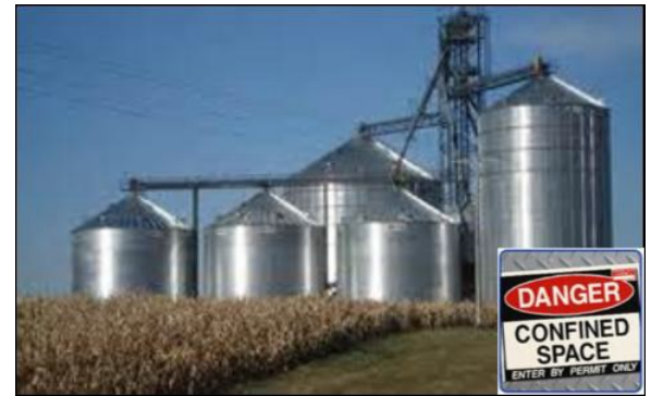
Figure 1. Excellent tools for storing and marketing grain, grain bins can also be a significant safety hazard. Knowing the safety rules and adding proper signage around bins can help prevent tragedies.
